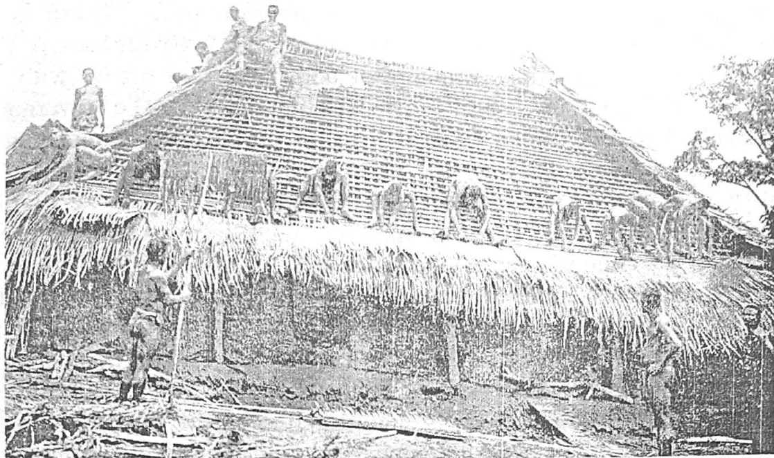
Plate 4: Thatching with palm leaf mats, among the Igbo people in the early 20 th century. An example of communal effort in community development. (Source: Basden, 1921)
